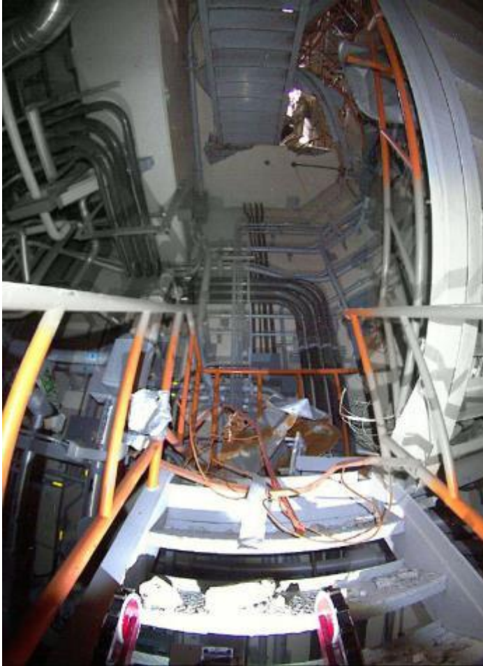
Stairs inside Fukushima-Daiichi plant occluded and impassible by conventional robots.
